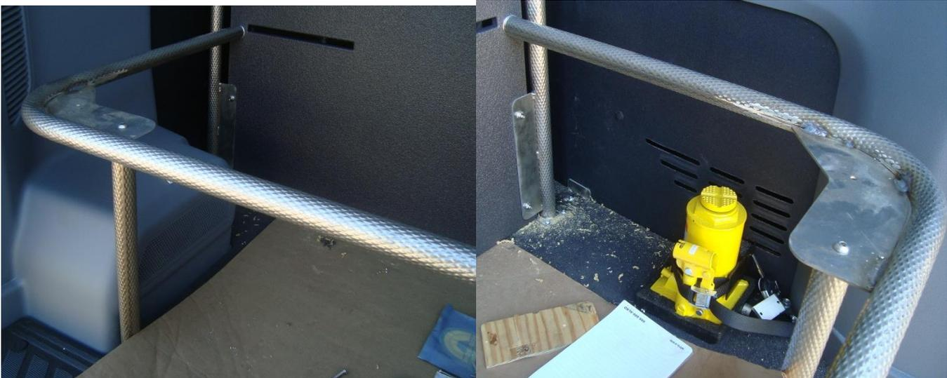
**Step 2** – Bolt the ends of the shelf perimeter tube to the lower partition panel using the 5/16"-18 Hex Head Bolts. These bolts are installed by reaching around the back side of the partition vertical tubes.
