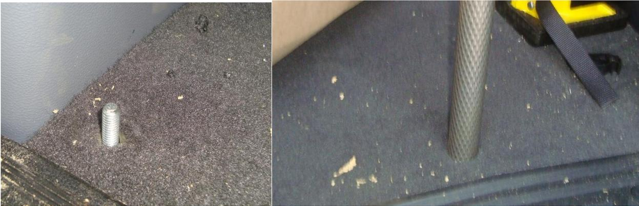
**Step 6** – Remove the 5/16” Bolts that were temporarily installed at the tops of the support legs and carefully place the shelf onto the frame. The “tabs” along the inner edge of the shelf must engage into the “slots” in the lower partition and the shelf must also rest against the top legs of the angle brackets. If there is to be only 1 shelf, reinstall the 5/16” Button Head Bolts through the shelf and frame tab and into the upper ends of the support legs.
